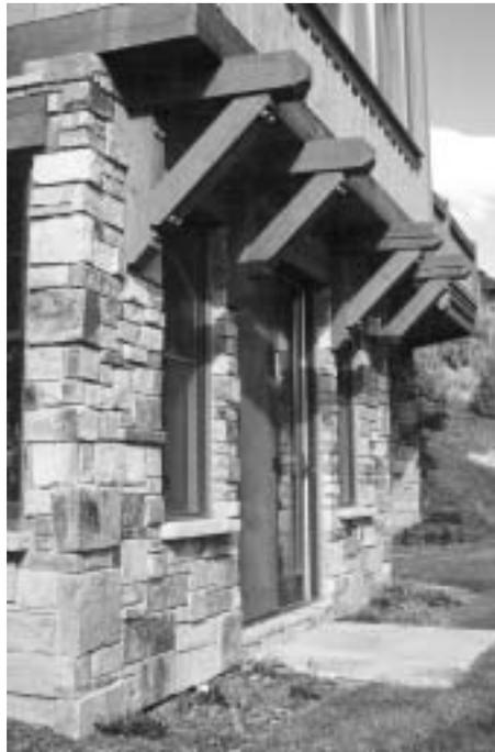
Figure 4: Structure should be expressed honestly, with apparent loads carried down to a stone or stucco base.
